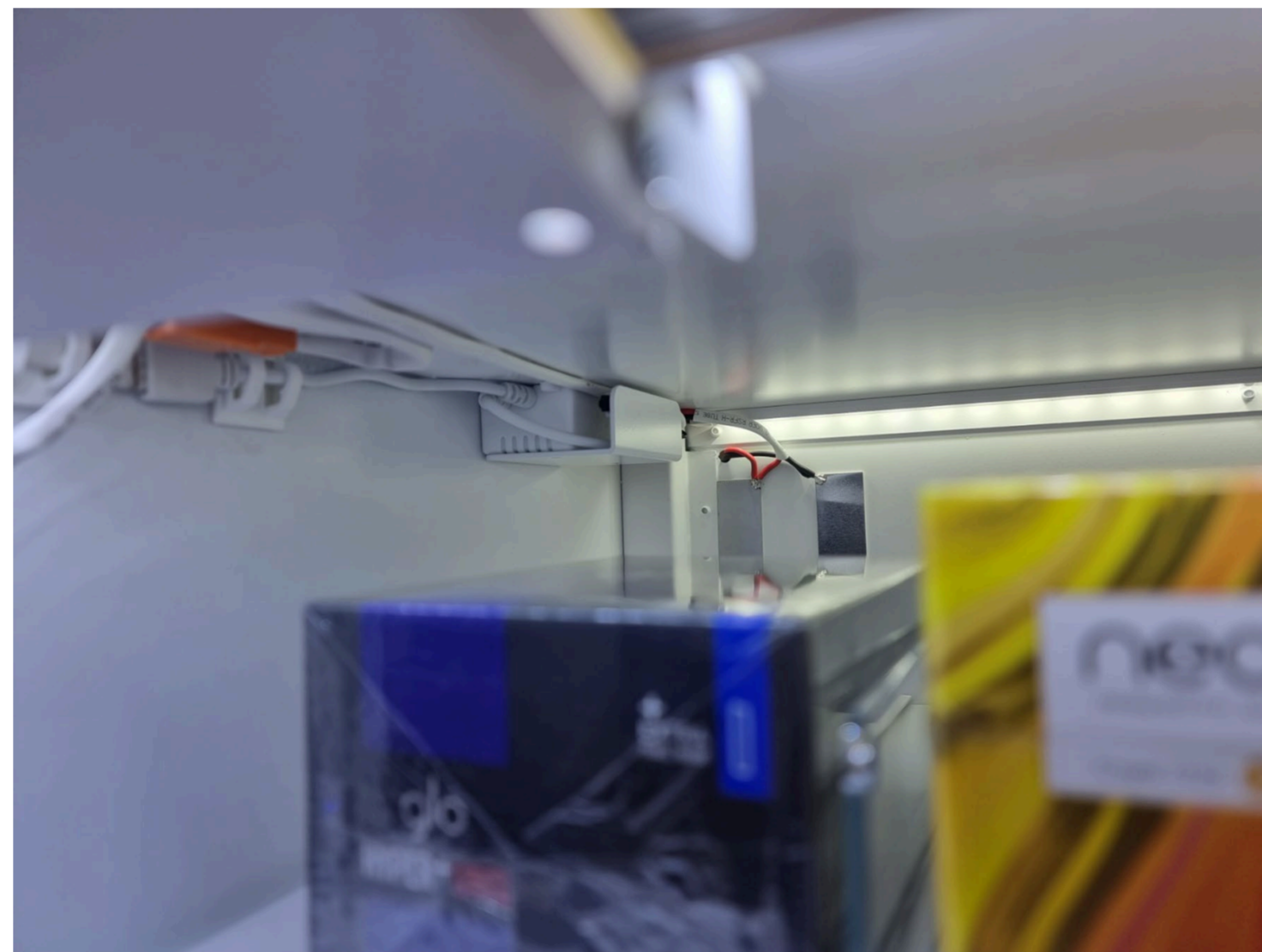
RGB Cables moved inside of the box
